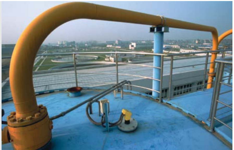
Silo roof with filler line, ventilation connector and ultrasonic sensor for measuring the filling level
